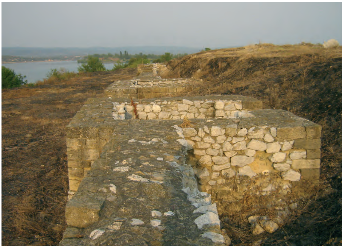
Fig. 14 Pontes – Fort, West gate
